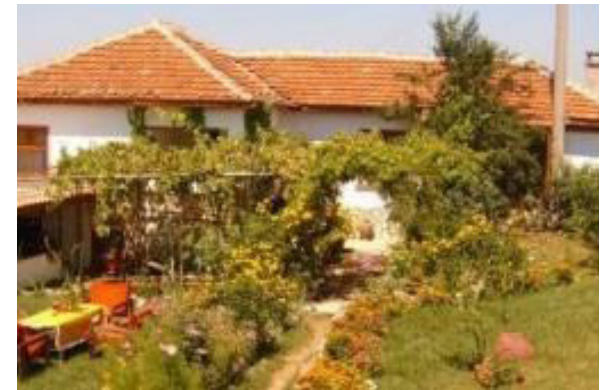
Residential and stable building, "Wild Farm", Gorno Pole, Bulgaria
